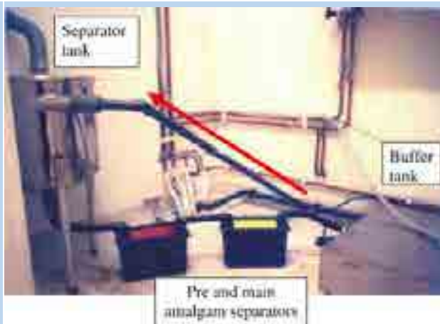
Photo 24: Amalgam separators from dental clinic, example of design. Source: (Hylander, Lindvall, & Gahnberg, 2006).
